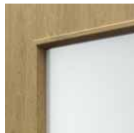
glazing bead with a glass panel
